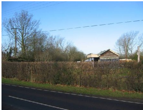
Old station building
