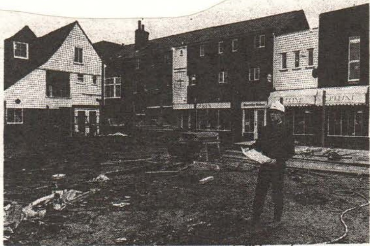
Builder's sub-agent Neil Fisher checks progress on the Waitrose site.
